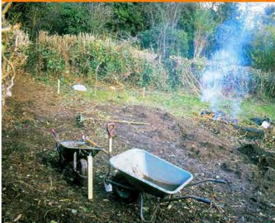
Flashback to last month...clearing the site, ready for action
