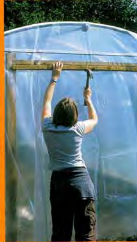
Fixing the polythene around the door frame with battens
