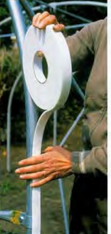
Fixing anti hot-spot foam tape to the outside of the hoops
