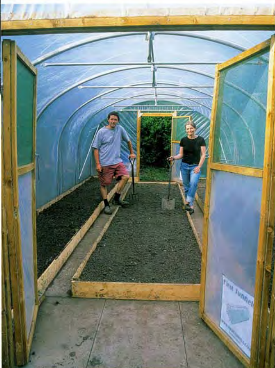
Phew – we've done it! The finished product with paths laid, beds dug and retaining boards in place
