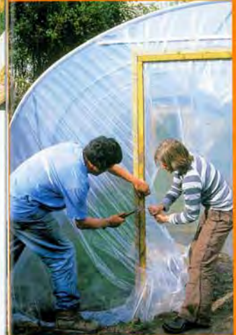
Pulling the polythene tight around the frame – one of the hardest parts of the whole job
