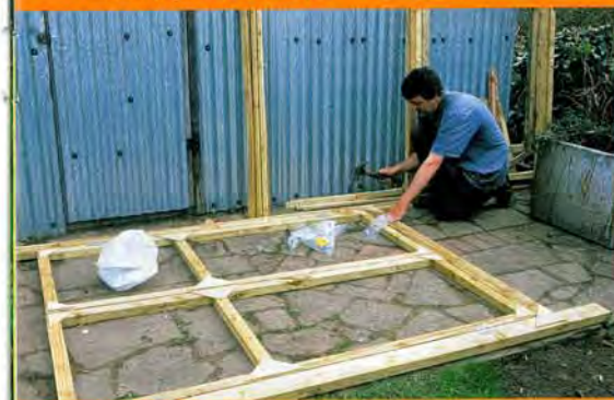
Assembling the double doors and door frame
