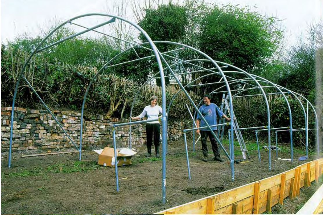
Laying out the polythene in readiness for pulling it over the frame – note it's a calm warm day!
