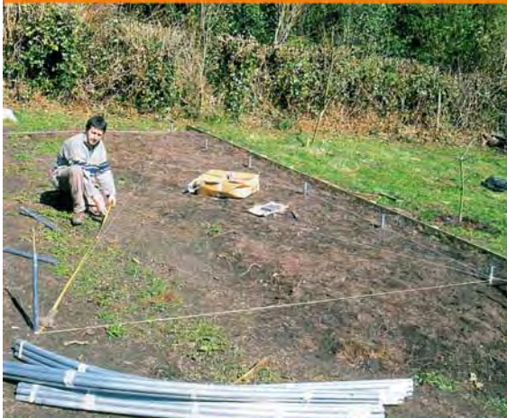
Using triangulation to check it's a true rectangle
