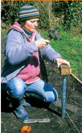
Sinking the foundation tubes
