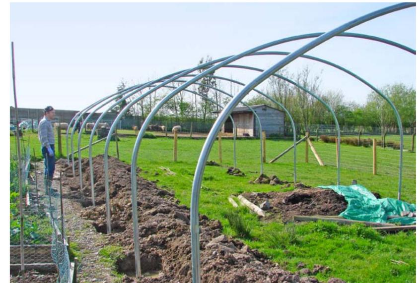
As you can see, much more earth was excavated to set the foundation tubes on one side of the tunnel than the other.
