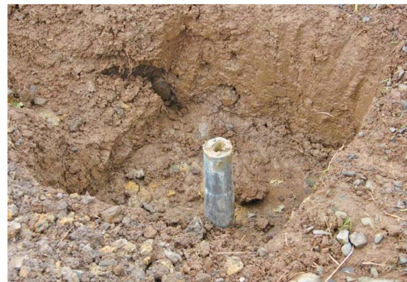
On the upper side of a slope, foundation tubes need to be set deeper than on the lower side.
