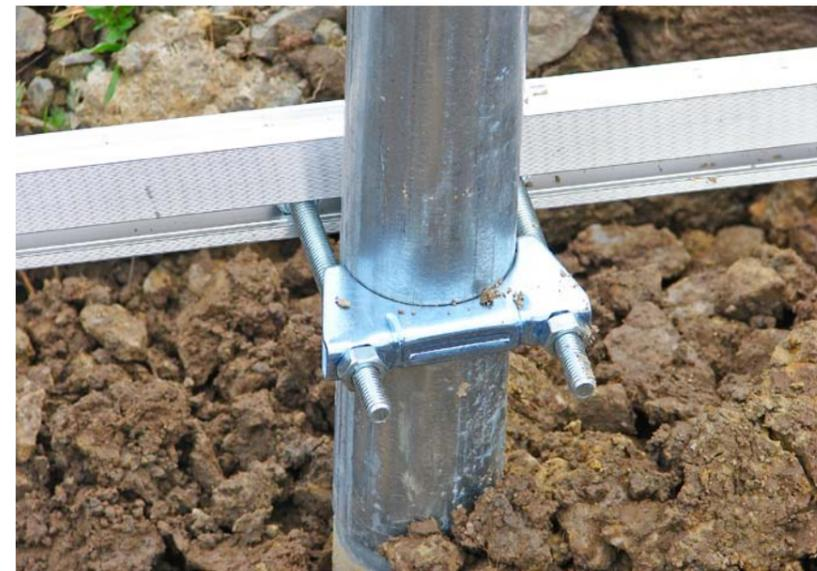
The entire rail assembly is clamped into place on the hoops.
