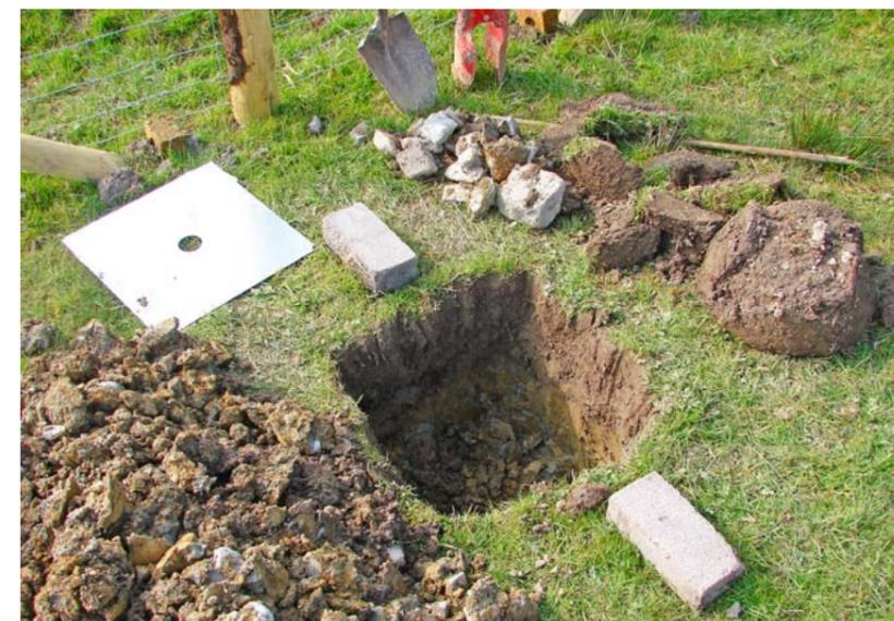
Holes are dug for the foundation tubes and their anchor plates at the points determined by using the '3, 4, 5' method and simple measuring.
